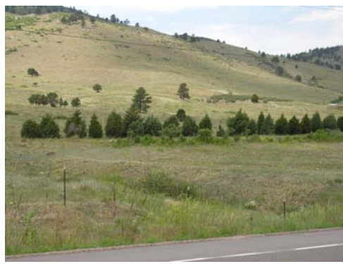
Figure 5 The Foothills snow fence has a row of shrubs in front of two rows of conifers. Note the set back distance.
